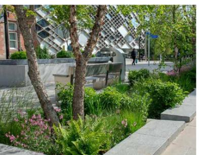
Figure 53: Raingardens with outlet kerb in stone
