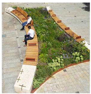
Figure 52: Raised planter with integrated seating
