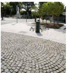
Figure 45: Clear paving transition, and use of traditional cobblestones to slow down traffic
